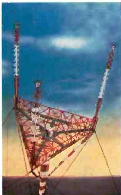
RCA designs and builds the equipment that transmits the TV signals.
