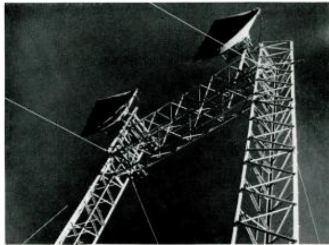
Western Union is installing a cross-country microwave system.
